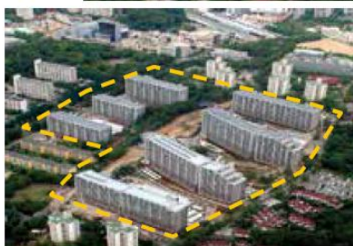
Reconstruction of a large condominium complex
