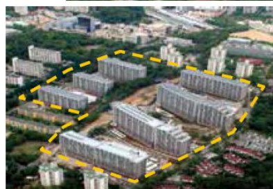
Reconstruction of a large condominium complex
